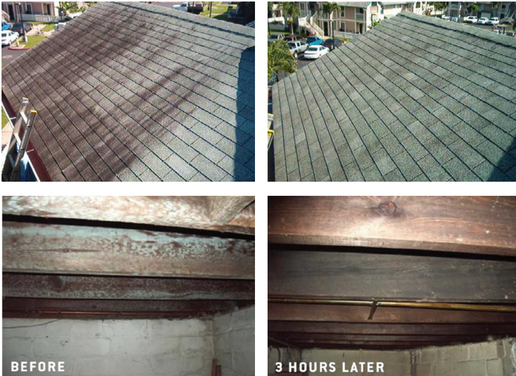
Picture 2: Mold remediation with PURStrike decontamination formula.
